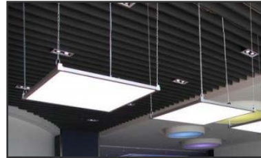
Option-2. Installation through Spring fastener
